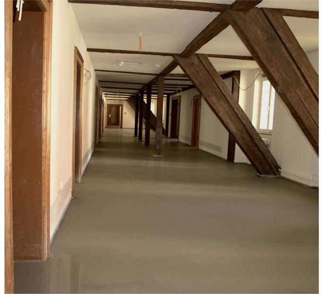
In this historical cloister area with a clinic operation UZIN NC 170 LevelStar was applied in different thicknesses on the most difficult substrates. The result is a perfect surface with optimal spread characteristics, and of course without any cracks.
