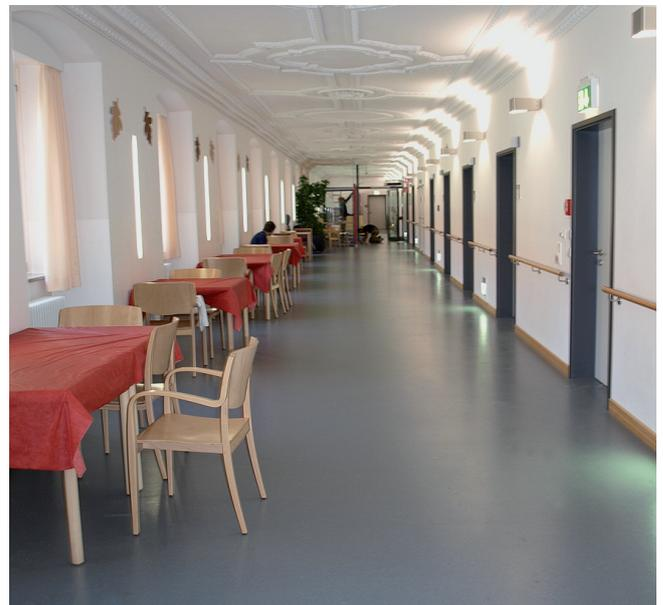
On other floors, stressed, highly-loaded floor coverings were laid on NC UZIN 170 LevelStar. The appearance is high-quality and there are no longer any corrugations or trowel marks with this premium levelling compound.
