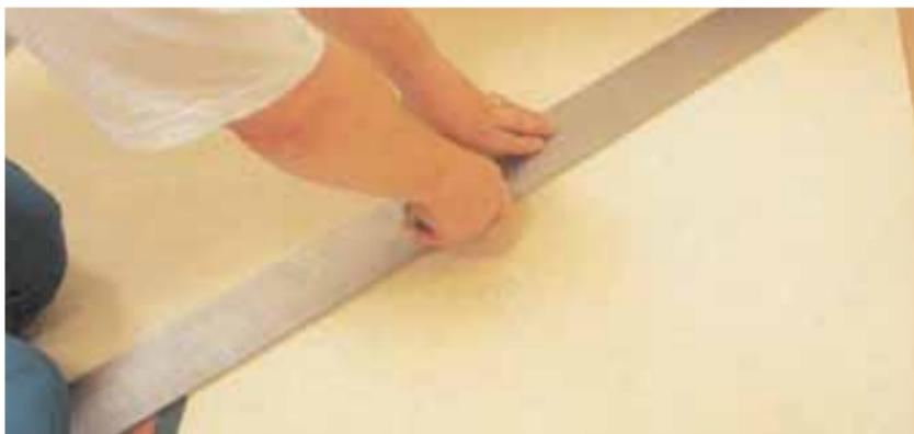
If the border is only a single surround of a contrasting colour then cut this piece approximately 70mm wider than the area to be fitted and scribe and cut off approximately 30mm along the wall, leaving about 40mm of overlap over the field colour. Cut this in as you would a normal seam, as described in an earlier section. The installation may look even more attractive if this seam is hot seam welded with a contrasting colour of welding cable.
