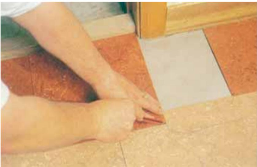
11. Cut all such edge tiles and place them and the full tiles still to be stuck on the adjacent tiles while fresh adhesive is spread in the border areas. Place the tiles and roll them thoroughly, using a hand roller or side of a hammer if necessary in corners.
