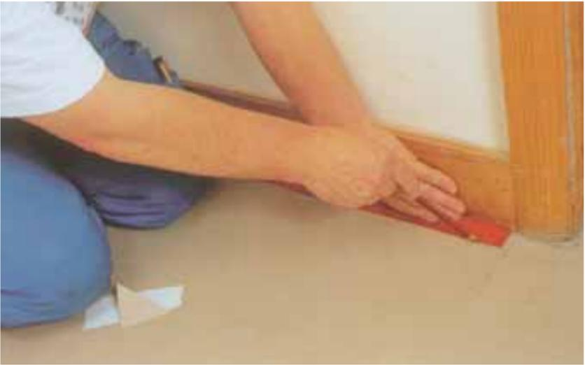
3. Use the same method to trace any objects such as WC pedestal, drawing a series of straight lines.
