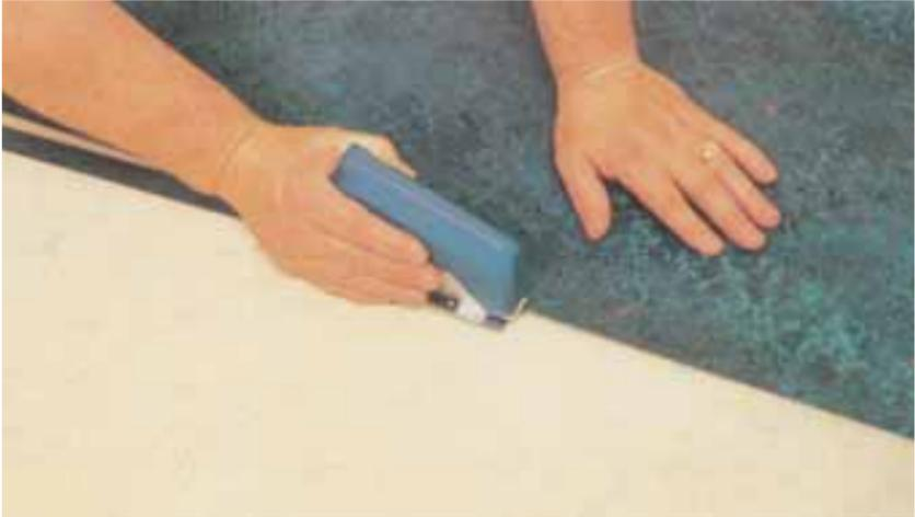
Cut the strip to be fitted against the wall 50mm wider than its finished width (i.e. cut to 700mm in this example). Butt this piece firmly against the field material, set the bar scribe to the full width of the total border pieces (150mm) and scribe to the wall as described in earlier sections.
