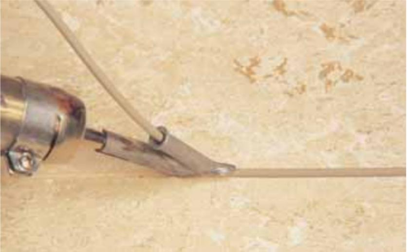
After the first 30cm check the weld is good by gently pressing the cable in the welded section from side to side. If the speed/heat/pressure combination is incorrect the weld will either come out or the cable will have melted over the sides of the groove, possibly with charred material either side of the groove. Below is an example of too hot a weld.
