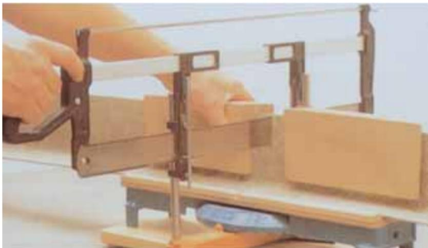
For pre-shaped coving, scribe internal corners for a mitred fit as described above and cut on the mitre block.
