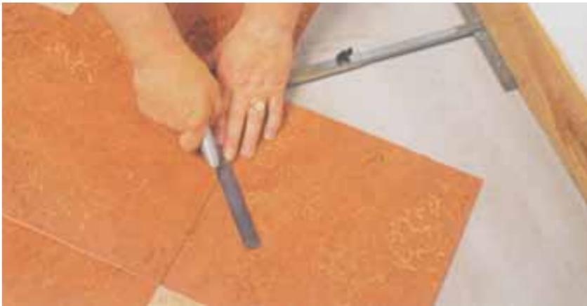
When all tiles have been cut to size and laid adjacent to the area they will occupy, spread the adhesive, lay the tiles and thoroughly roll them.
