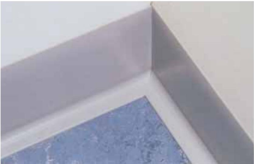
With set-in coving, the toe of the first length is mitred before being stuck and the scribing of the second length continues down over the toe so that a fully mitred joint results.
