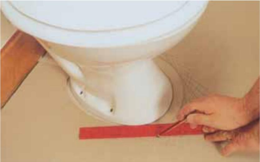
Another method is to let the paper ride up all the sides of the pedestal, making numerous relief cuts to enable it to do so, then draw a firm pencil line on the paper at the bottom of the relief cuts, pressing the pencil into the angle at the bottom of the pedestal.
