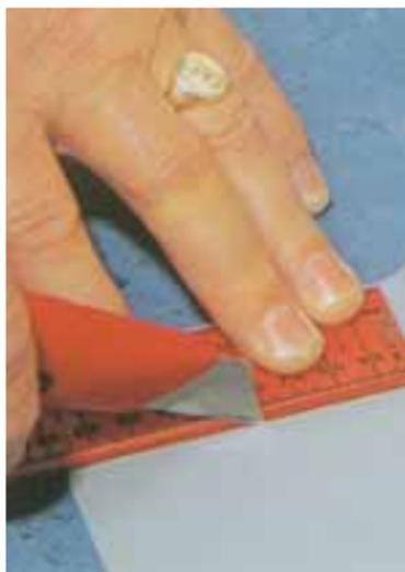
Push the knife into the swing at two points on this line. This will show as two white marks on the front of the coving. Cut along this line and also along the pencil line on the toe. Join the two cuts with a curved freehand cut.
