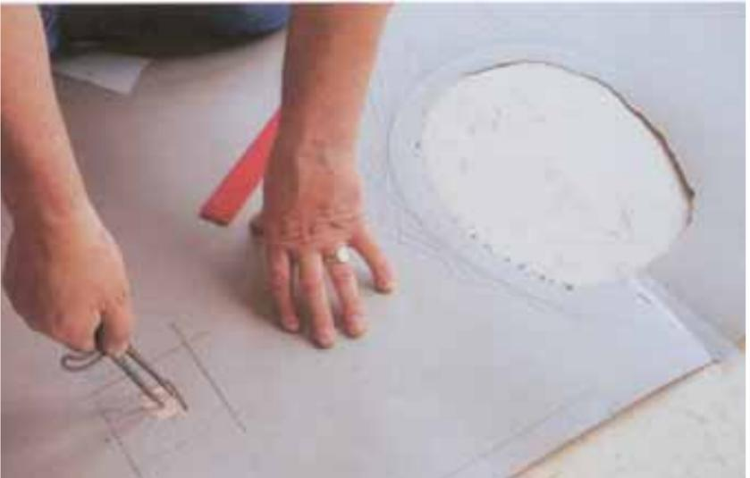
After checking that all scribe marks have been transferred, remove the paper template.
