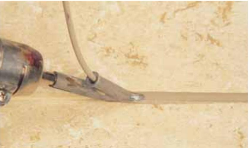
For the last few cm against the wall behind you, take the cable out of the feed, trim off at the end of the section you have welded and chamfer it down in the grout. Starting at the wall, weld over the chamfered section, applying pressure. Trim off.
