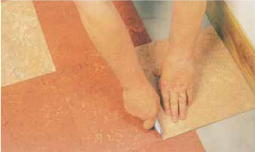
10. For fitting to door frames, etc, use the same principle of fitting the tile to be cut in the position of the last full tile and marking each change of direction of the door frame by using a bar scriber set to 500mm (or the tile size), or a rule, before cutting carefully. The position of a pipe can be marked and cut in the same way.
