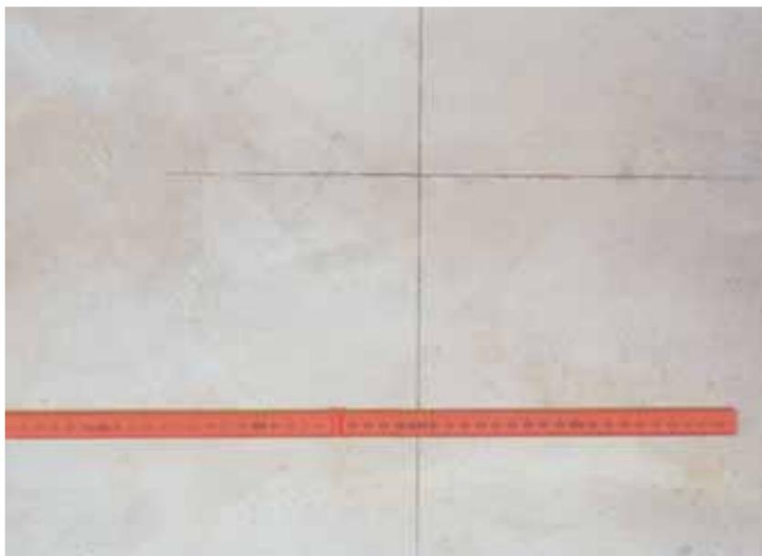
Cut the field material so that it overlaps this chalk line by about 50mm all round. Seam sheets in the normal way then pull back half at a time and spread the adhesive exactly to the chalk line, leaving the 50mm unstuck. Put the field sheets into the adhesive and roll thoroughly.
