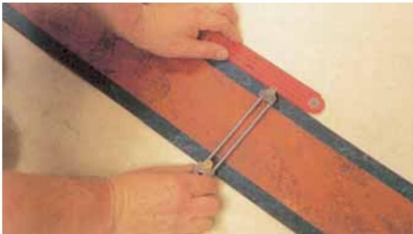
Remove this piece and fit the other border pieces into position, from the inside outwards. The scribed piece will fit neatly against the wall. Once the fit has been checked, remove the pieces and spread adhesive between wall and field, rolling thoroughly once the border pieces are in position. Clean off any surface adhesive while it is still wet. Mitre corners with the help of a straight edge.
