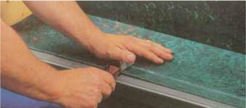
Use an adhesive with a high initial tack for linoleum. For vinyls use an acrylic adhesive with a lift and drop double stick method. No adhesive is put under the vertical part of the nosing.
