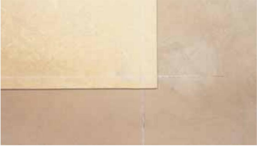
Cut the border strips along the length of the material, especially if it is linoleum. If cut across the width - which is often tempting as it could reduce scrap - the strips will curl and dome. For strips up to 30mm wide, the Forbo Trimmer is ideal. Cut wider strips with a straight edge.
