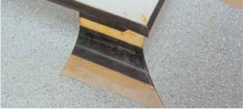
Trim the top of the coving to the chalk line on the wall or check it will fit into the capping strip, if one is being used.
