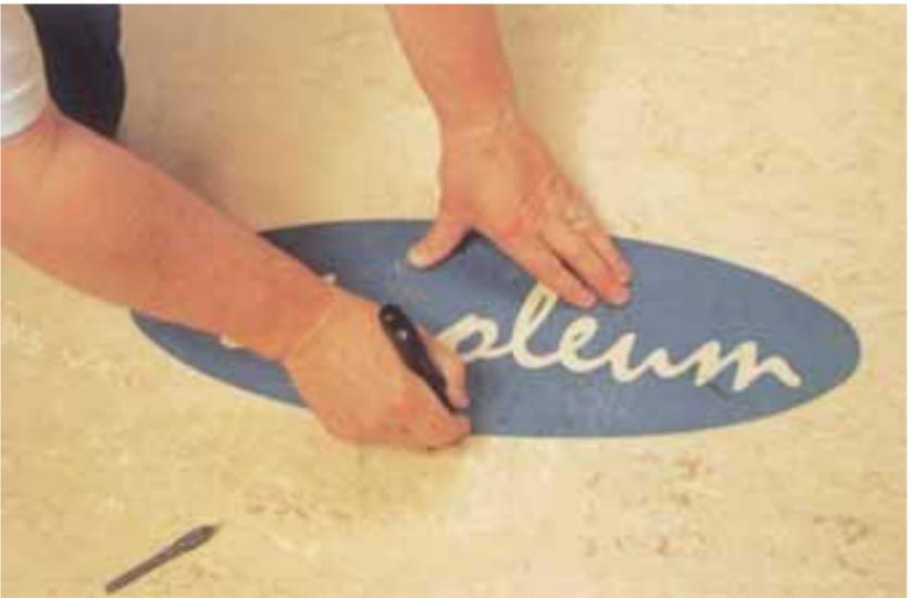
Pre-cut designs are almost always pre-assembled and held in place with clear tape. This should be removed immediately after rolling so that if any adjustments are necessary these can be made before the adhesive starts to cure.
