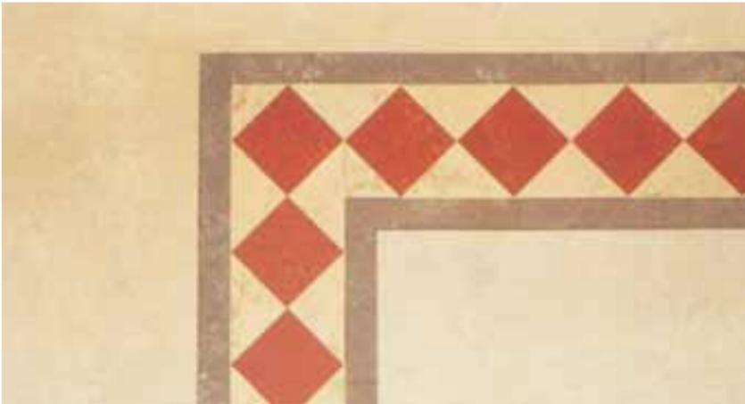
To fit the material between the border and the wall first scribe a piece of material about 50mm wider than the greatest distance between the outer edge of the border and the wall. Set the bar scribe to about 25mm, butt the material against the wall and scribe and cut to the wall. Fit the inside edge to the outer edge of the stuck-down border, using the over and under scribe.
