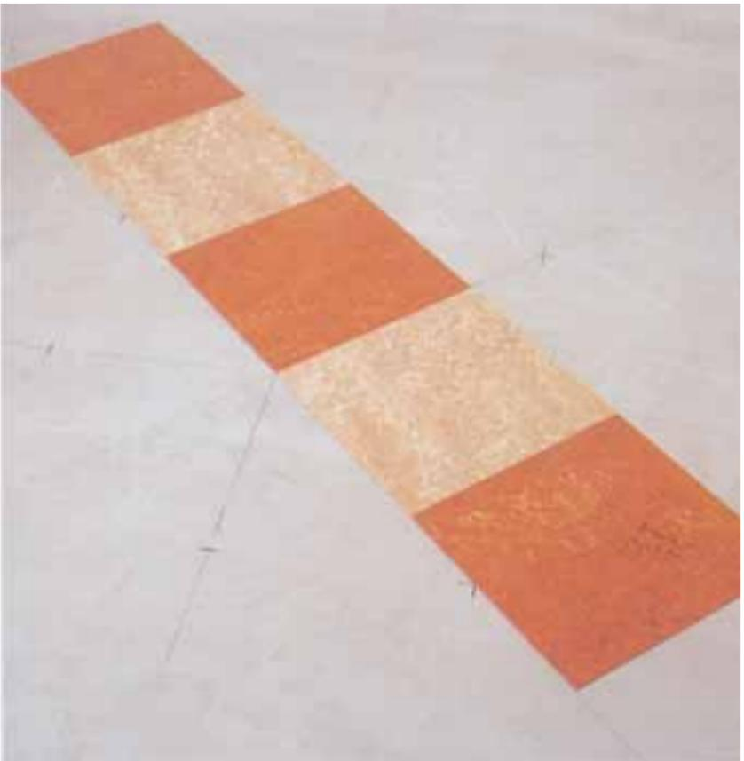
Once again, the key and first row tiles are all important. When balance has been achieved and the first row tiles correctly stuck, lay the field tiles and roll them before the adhesive has set off. An extra check on accuracy is that the points of the tiles should fall precisely on the centre lines drawn at rectangles to the walls, as shown below:
